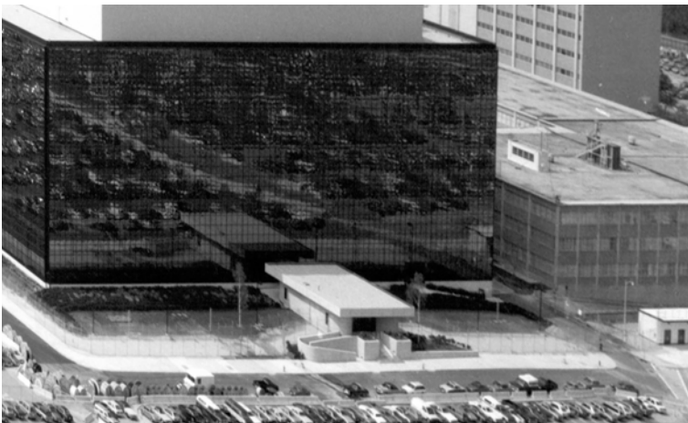
NSA headquarters Fort Meade, Maryland, US, 2013
